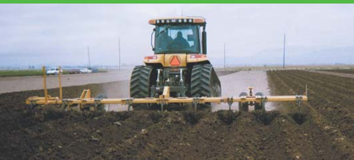
Final Pass - Perfect Positioning
